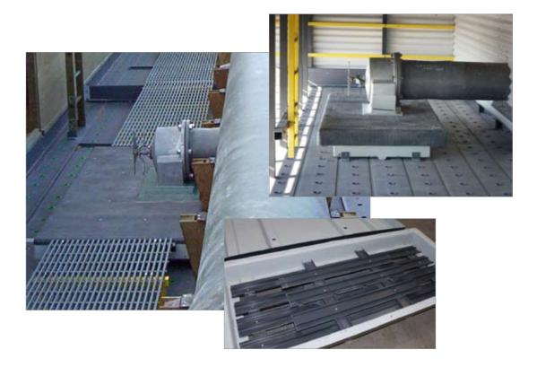
The Midwest Towers water distribution box is designed, engineered and manufactured of strong, lightweight, non-corrosive fiberglass reinforced plastic. It is perfect for all crossflow cooling tower applications. It helps deliver a uniform flow of water from the flow control valves into the hot water basin of the cooling tower. This is essential for optimum thermal performance.
