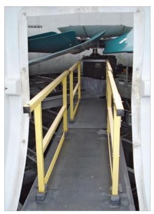
The strong, light fiberglass panels or grating can be custom-designed for the best fit around mechanical equipment for maintenance and service.
