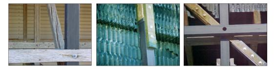
Midwest Cooling Towers pultruded fiberglass structural shapes allow you to replace deteriorated wood columns, beams, and decks on your cooling towers with strong, lightweight, rot-resistant fiberglass.
